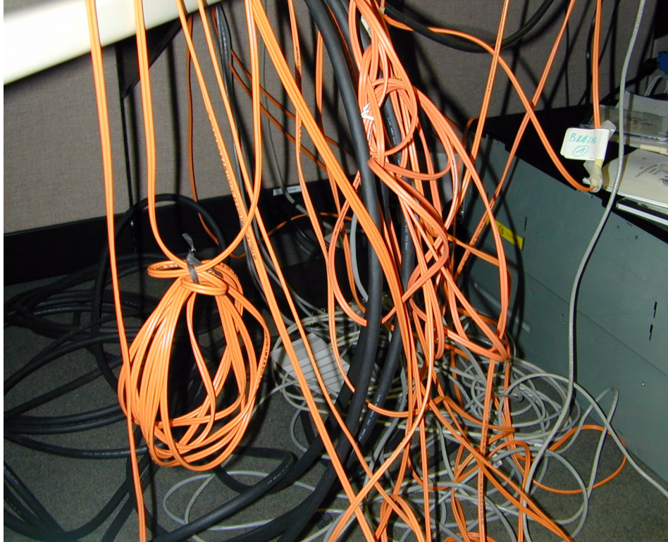
Figure 4-2 Messy cabling, no cabinet, and no cable labels
